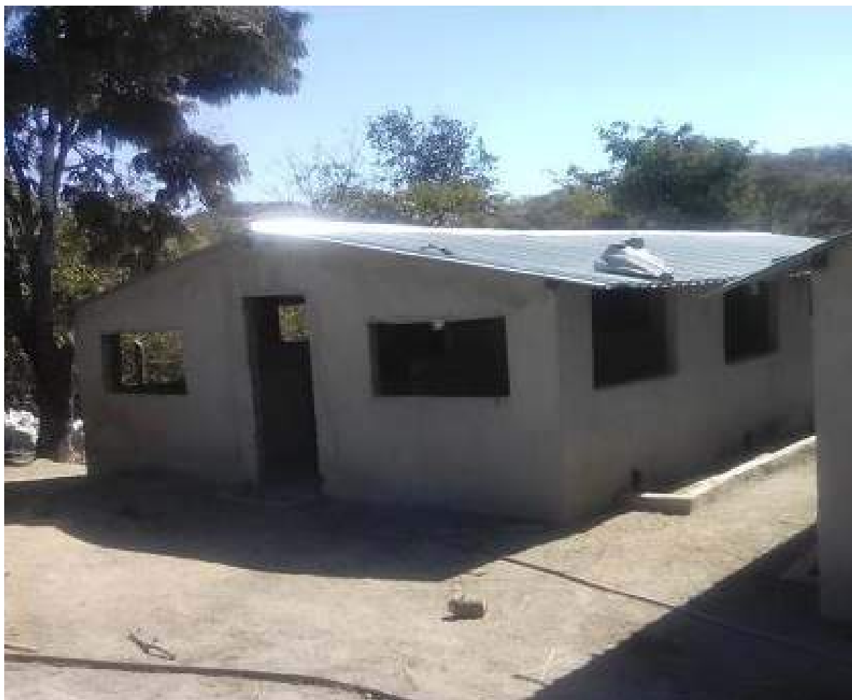
Figure 6-3 Cement plastered brick walls
