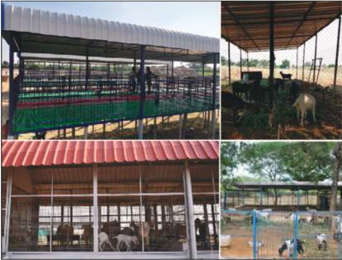
Figure 6.12 Steel bars/Fence Roofed goat pens
